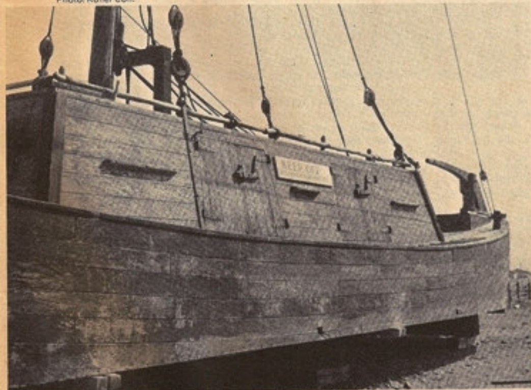
A close-up of keelboat superstructure showing the cargo housing.
